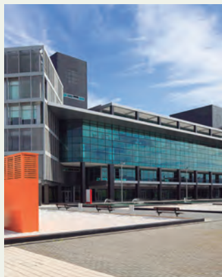
Andalucia Technology Park. Offices of high energetic efficiency. Spain. ECOi
