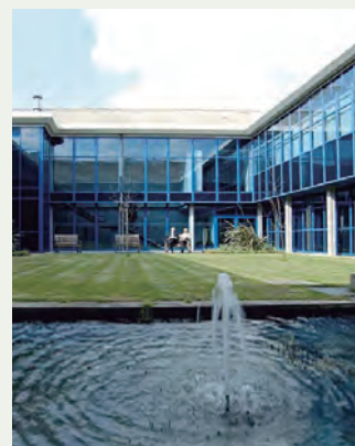
NHS Canford house clinic, Bournemouth, UK. VRF
