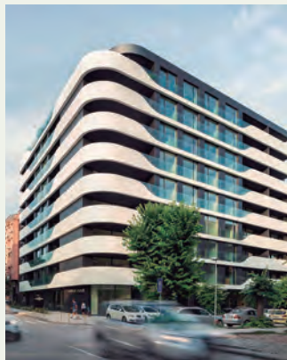
Bulgaria's stand-out residential building with efficient HVAC solution. Aquarea
