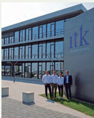
ITK Engineering GmbH. An innovative office building located in Germany. ECOi - PACi
