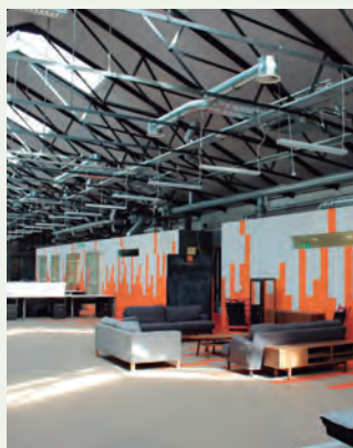
Zalando's solution for its warehouse office conversion at Grand Canal Quay, Dublin. ECOi
